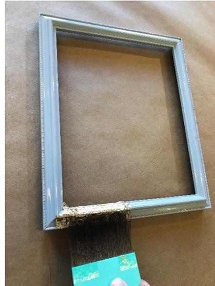
All sizes can be applied by brush, roller or sprayer. You want to apply the size as thinly and evenly as possible. Avoid pooling in corners and creases. For water based size which sets up quickly, it's important not to over brush the size as it will leave brush strokes. When the size reaches the proper tack you are ready to gild.
